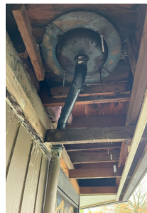
5. Unrelated to the January water break, but in need of water-damage repairs nonetheless. Rusted out “roof sumps” need to be replaced and rotted soffits repaired.
